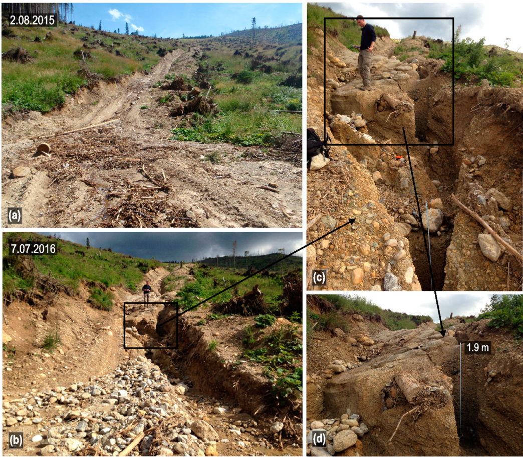
Figure 4. A forest road in the Lejowa Valley 1 year after construction (a), 2 years after construction: transformed by a rainfall event (b). Eversion kettles developed after the rainfall event in 2016 (c). The deepest (1.9 m) eversion kettle within the studied roads developed after the rainfall event in 2016 (d).
